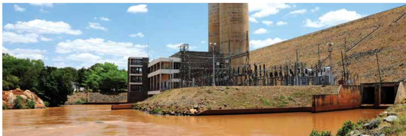
Masinga Power Station in the 7 Forks Cascade. It holds approximately 2 billion litres of water making it KenGen's largest dam in the Eastern Hydros area
