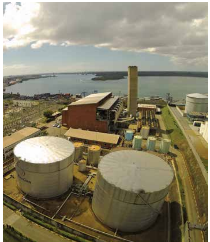
Aerial view of the Kipevu III Power Plant. KenGen produces 15% of its generation portfolio from diesel engines.
